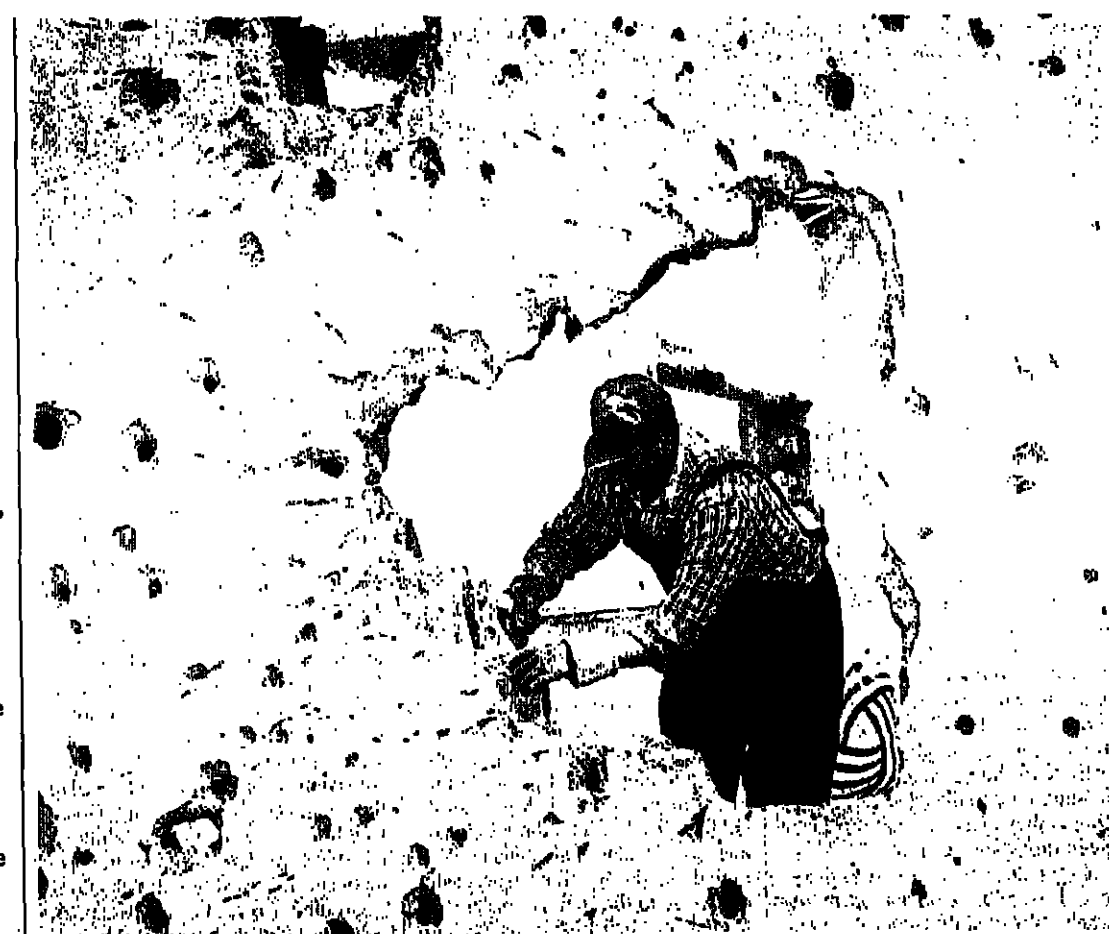
A man begins repairs on his house in a once front-line suburb in Sarajevo. PHOTOGRAPH BY DANILO KRSTANOVIC
